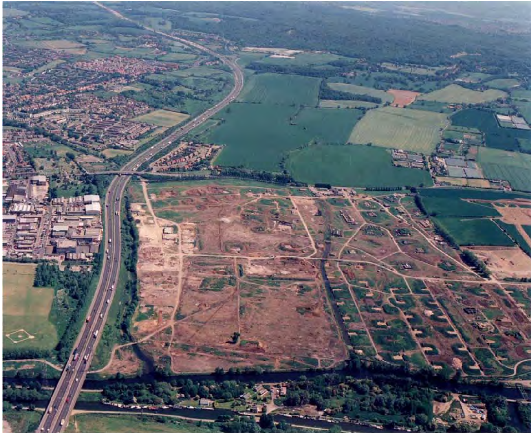
An aerial picture of the South Site after the site was first cleared.
