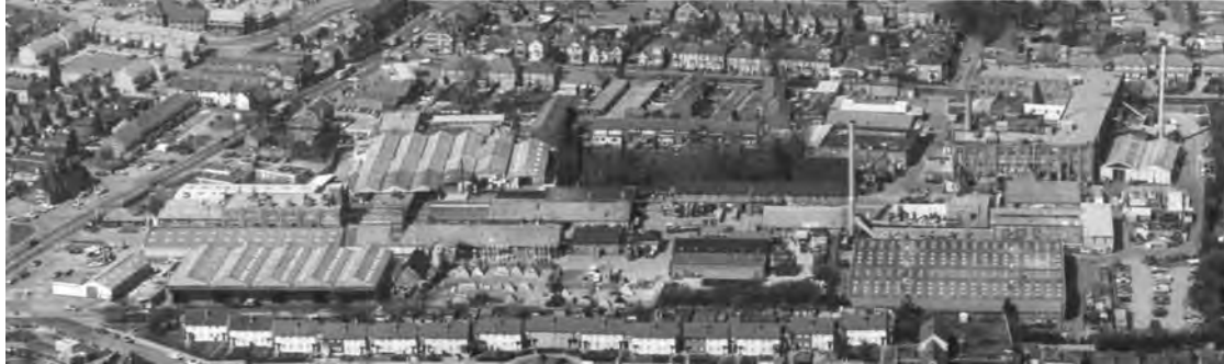
The factory complex in about 1974.
