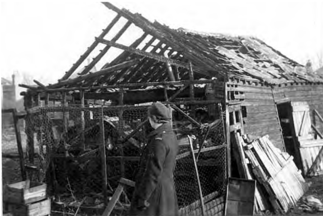
Rear of 100 Honey Lane. Damage to storehouses [Carter]
